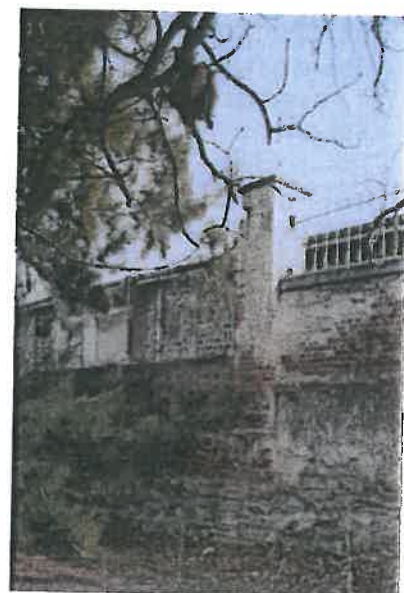
Lower level view of perimeter wall showing deterioration due to rising damp
