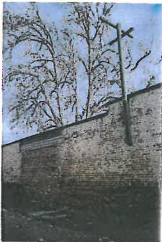
Perimeter masonry boundary wall With timber line mast.
