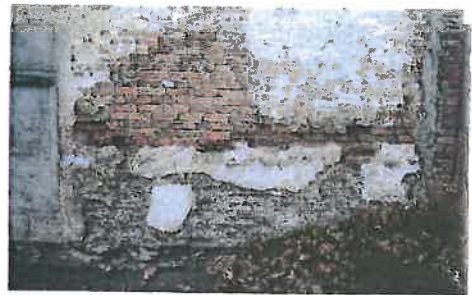
Wall detail showing rising damp, salt deposits and break down of masonry.
